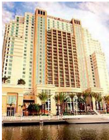
TAMPA MARRIOTT WATERSIDE (600,000 SF)
